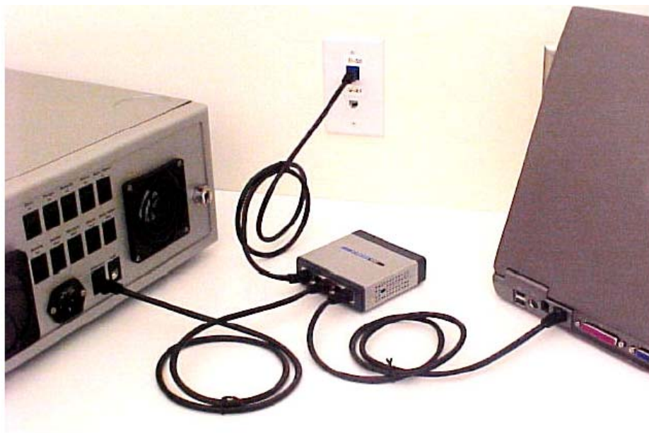
Figure E-9: Instrument and computer connected to LAN via Ethernet switch
